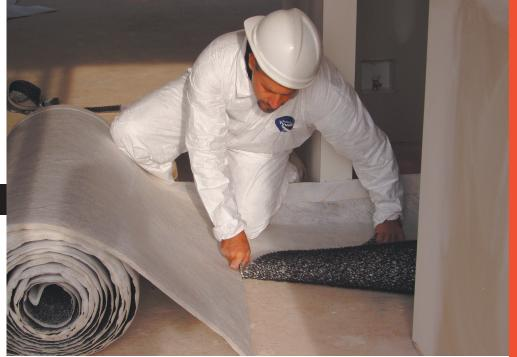
AccuQuiet<sup>®</sup> C40 is a polypropylene monofilament mesh, molded in a "Cuspated" configuration, and bonded to a lightweight water-tight technical membrane. The cuspated configuration of AccuQuiet<sup>®</sup> C40 yields enhanced acoustical performance properties, with minimal sacrifice in deflection characteristics.
